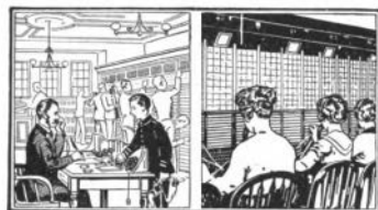
Early Telephone Exchange
