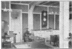
BEAVER BOARD is used in thousands of commercial buildings. This is the office of the American Mfg. Co., Clio, Mich.
